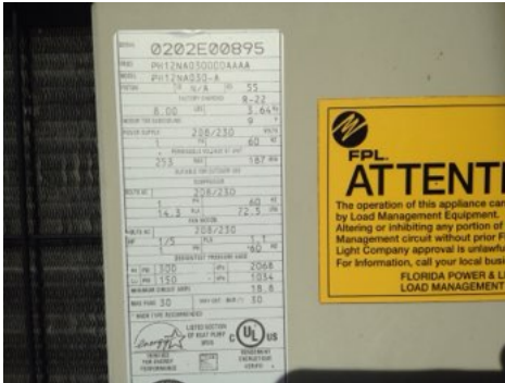
Condensing unit label. Manufactured in 2002.
