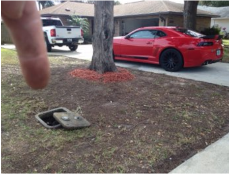
Main water shutoff is in here
