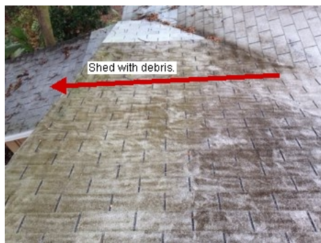
Mildew should be cleaned. Shed is on the left with the debris causing leaks.
