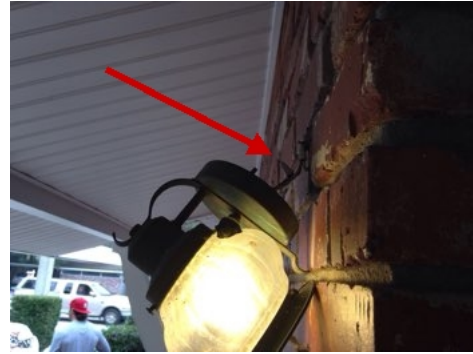
Exposed wires.
