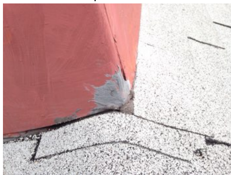
Covered flashing
