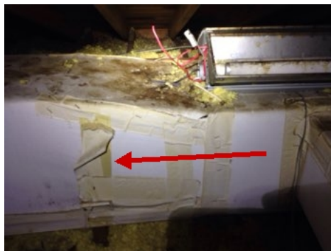
Air escaping here. This is near the attic access in the hall.
