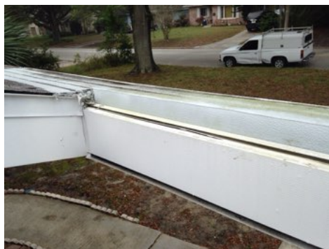
Exposed wood in here. Getting wet.
