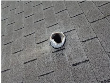
Vent pipes should extend 2-3 feet above the roof line.
