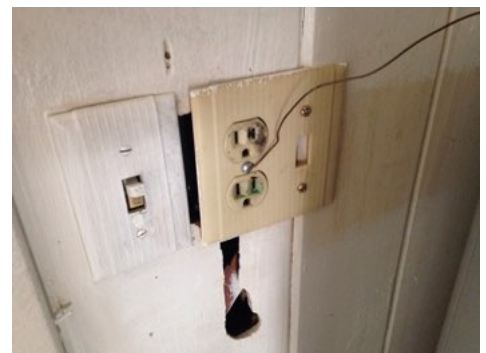
Scorched outlet near water heater
