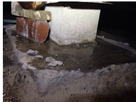
Leak under shower in master bath
