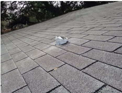
Vent pipes should extend 2-3 feet above the roof line.
