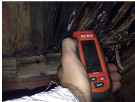
Moisture damage near tub in hall bath. Tested dry.
