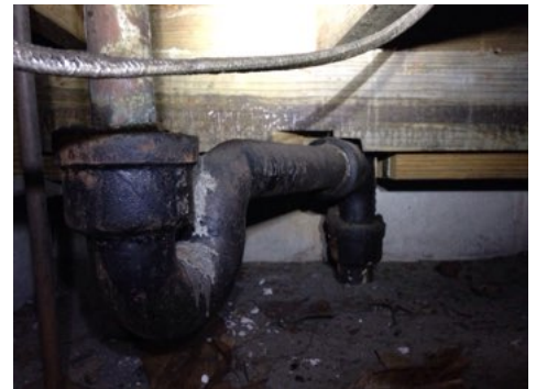
Cast iron waste line at master bath toilet and sink.
