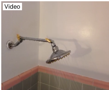
Shower head leaks when in use.
