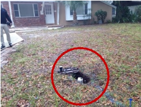
Main water shutoff is in here.
