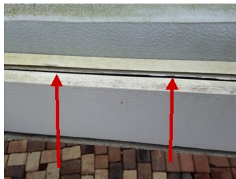
Gap in aluminum material.
