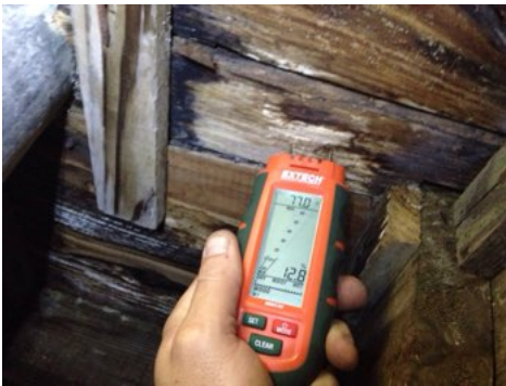
Moisture staining near toilet in hall bath. Tested dry.
