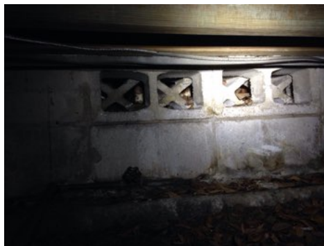
Missing screens in the front. Also these are blocked.
