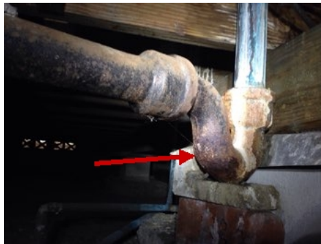
Leak in drain line at master bath shower
